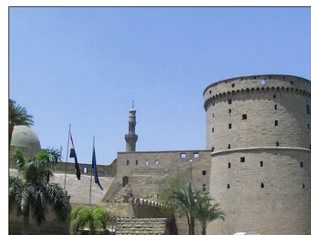
Part of the (Crusader style) wall around the Citadel
